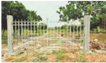
The Project's main gate under construction.
