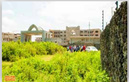
Ronald Ngala Utalii college & 5 star Hotel. Construction in progress
